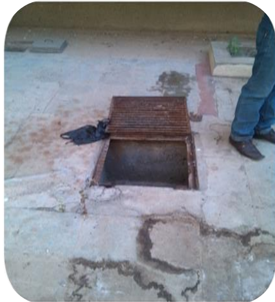
Uncovered underground sewage system & leaking sewage water- DH Bhuj, Kutch
